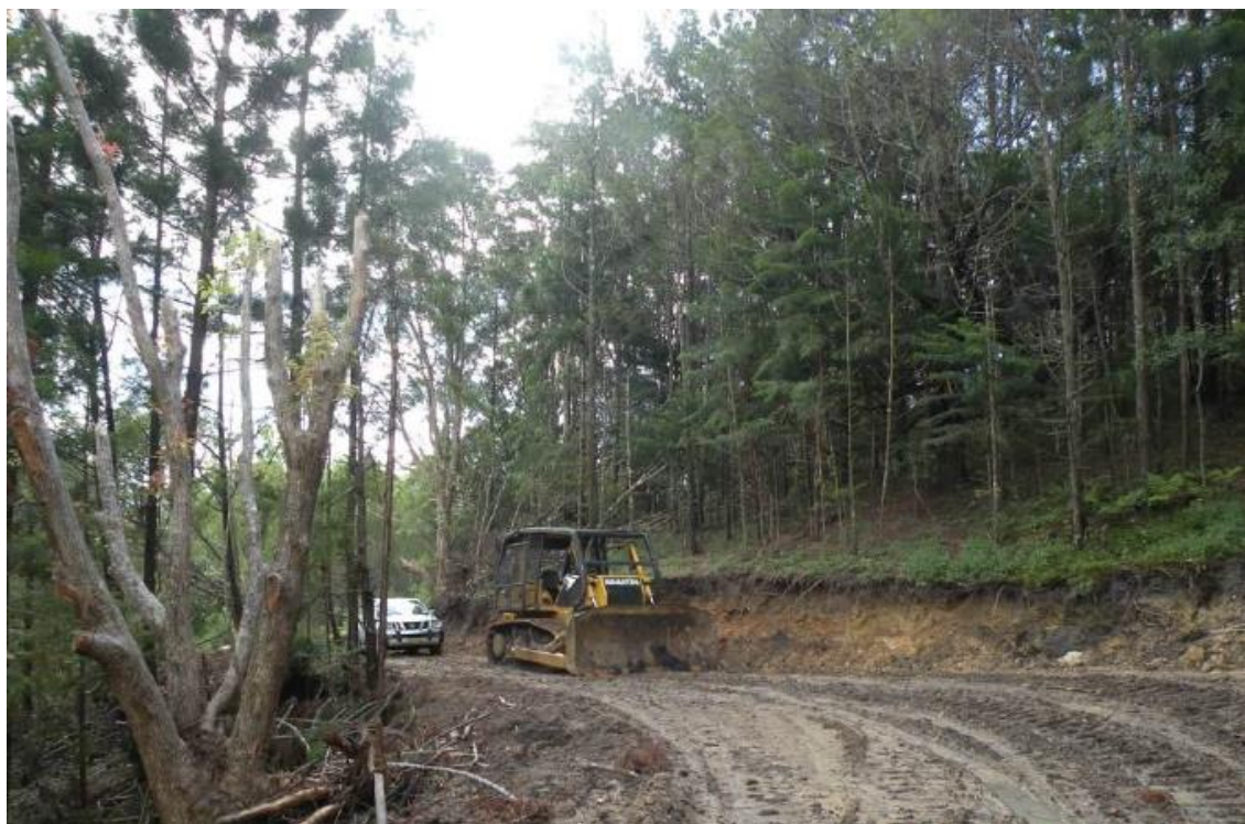
Photos showing construction of logging access roads which give rise to potential sedimentation and erosion concerns.
